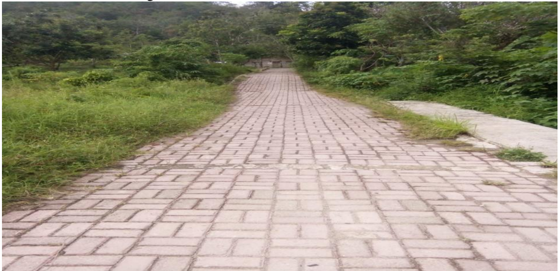
Gambar II. Jalan Paving Blok
