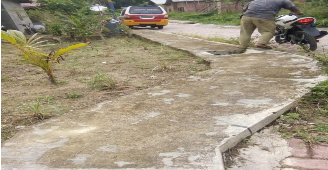
Gambar IV. Drainase Tertutup
